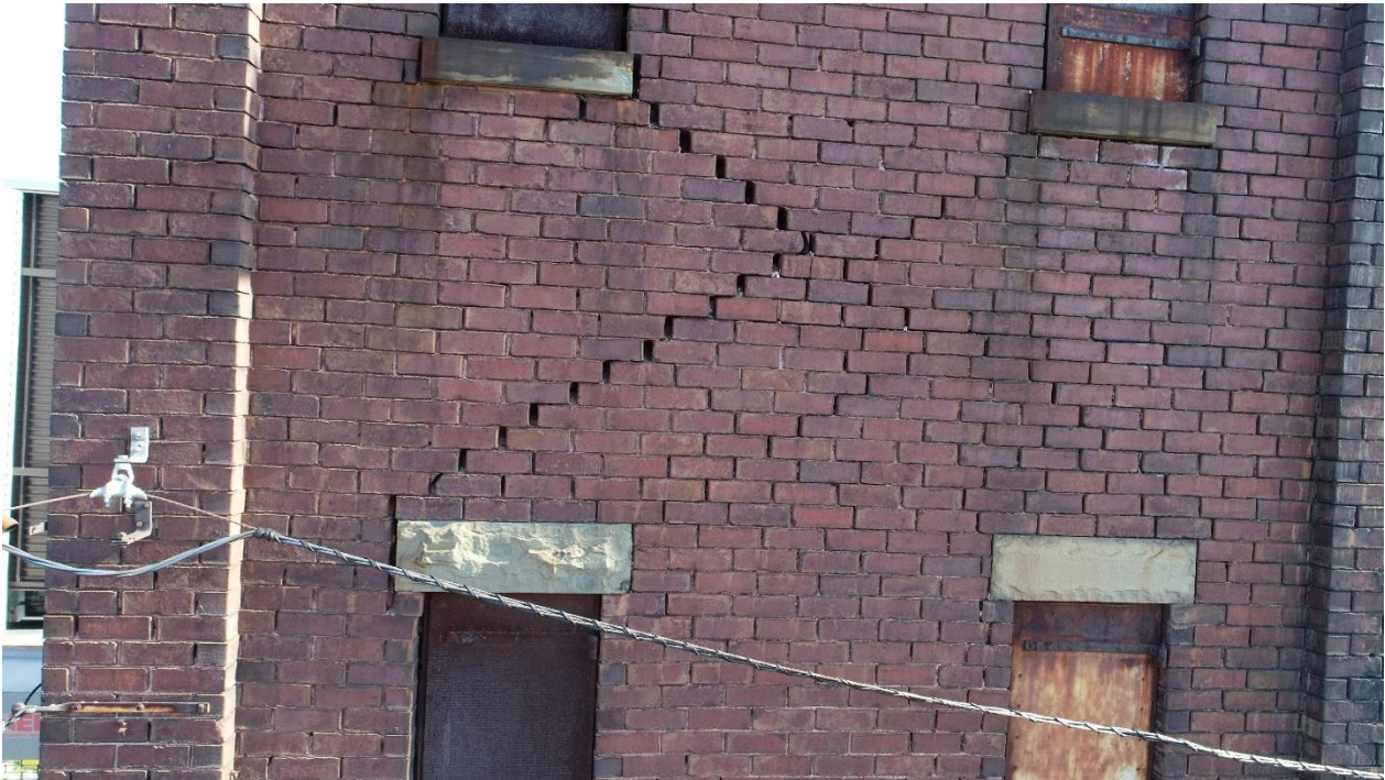
General Exterior Conditions Photographs Taken August 2019
