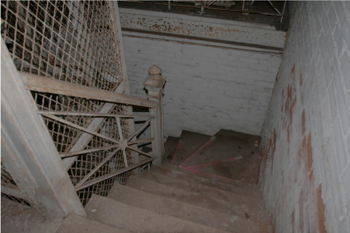
Interior Photographs Taken 2014
