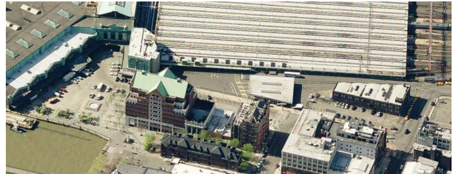
Aerial View showing Warrington Plaza / Hudson Place
